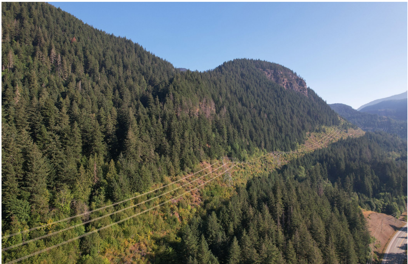
Photo 10. Transmission line near Yale.
